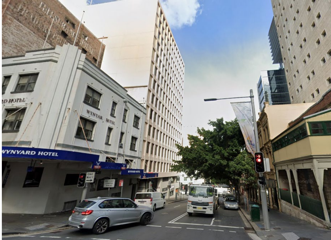
surrounding commercial development viewed from Erskine St facing west
